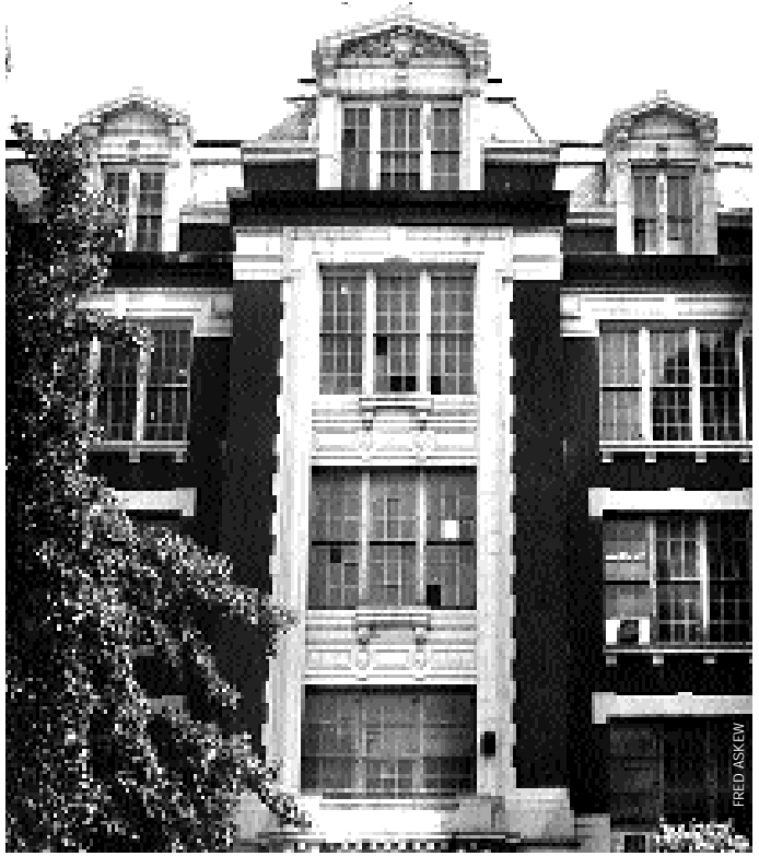
ABANDONED: The old school building at 605 E. 9th Street had been empty since the CHARAS/El Bohio Community Center was evicted in 2001.
